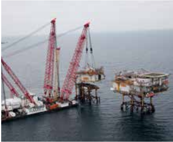
Removal of platform K10-B (courtesy of Wintershall Noordzee B.V.)
