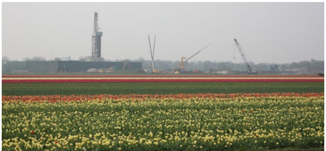
Injection/production location during the drilling and construction phase in the Bergermeer (courtesy of TAQA energy B.V.).
