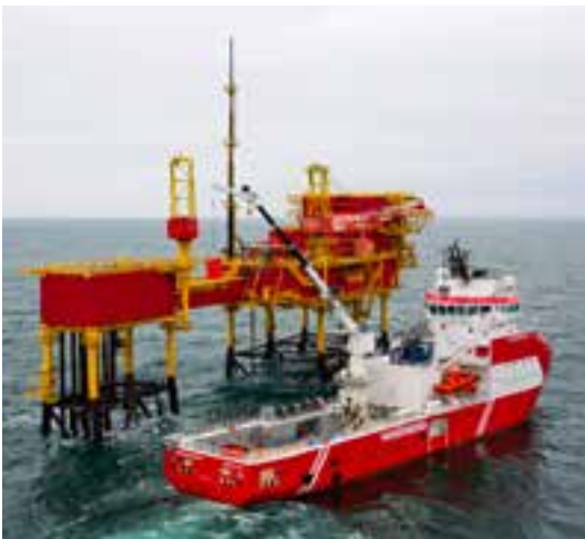
Kroonborg walk-to-work maintenance vessel (courtesy of NAM B.V.)
